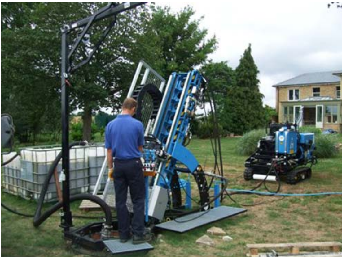
Geodrill 4R rig positioned on the drilling chamber with Power Unit.
