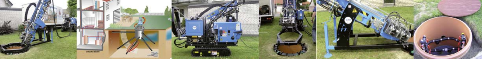
Jobsite Bruges/Belgium: 5 Apartments - 5 Drilling chambers with 200 m heat pipes each
